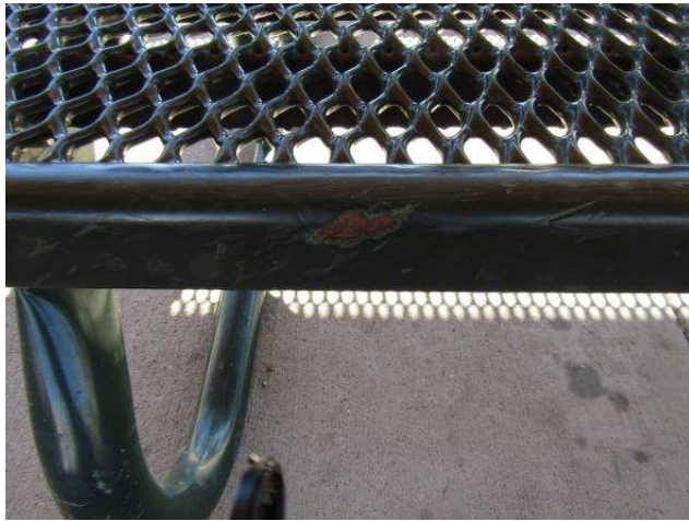
PVC damage on Table
