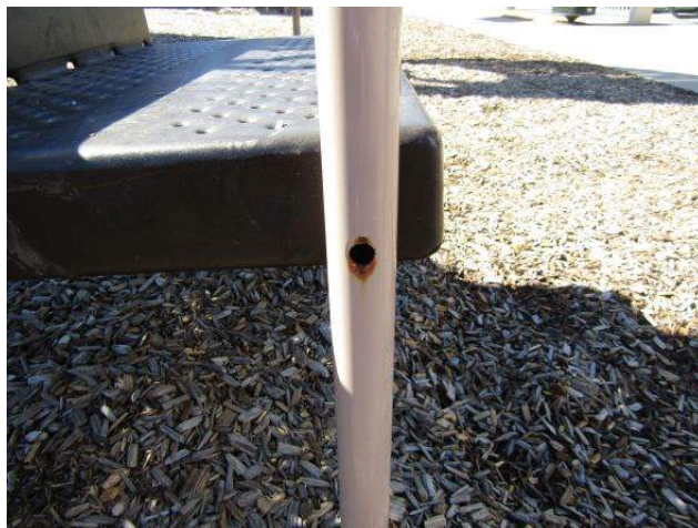
Transfer Station Missing bolt (Replaced during inspection)
