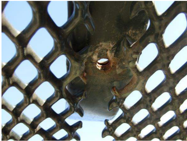
Shade Bench Missing Bolt
